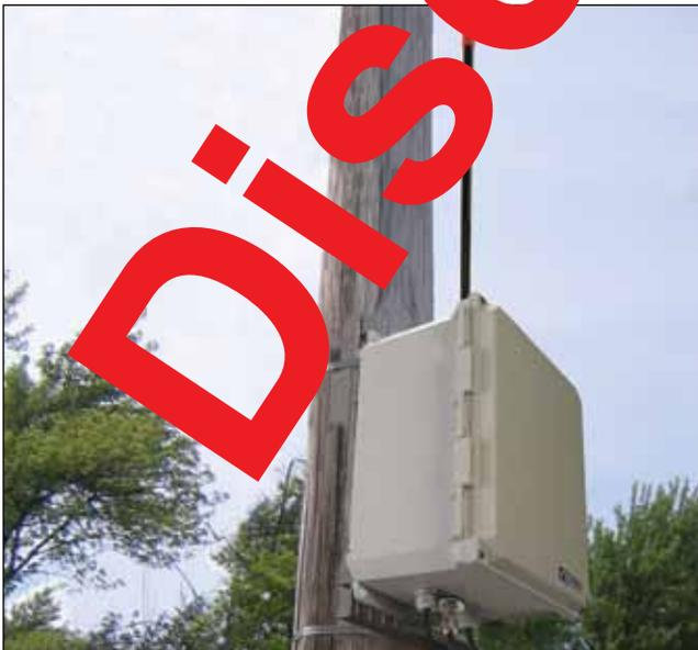
OM-AMPOLEMNT10 optional pole mount kits are 14 gauge (0.075") galvanized steel with 48" SS pole clamp and includes #10-32 SS screws, washers and lock nuts.
