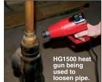
HG1500 heat gun being used to loosen pipe.
