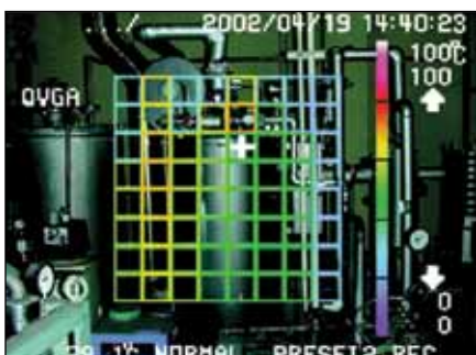
For the temperature control of boilers
